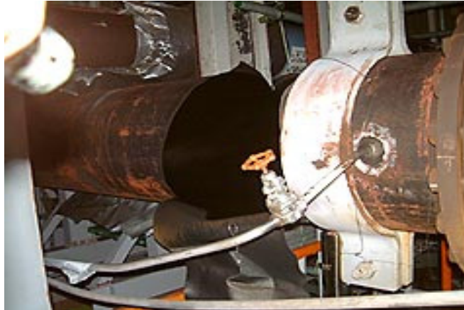
Figure 2. A recent pipe rupture accident occurred at the position just after a flow-meter with an orifice-typed device, reported in 2004 [16]
